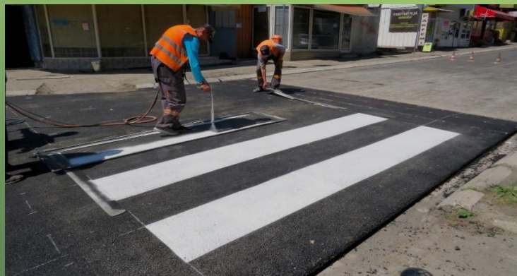
Raised pedestrian platform
