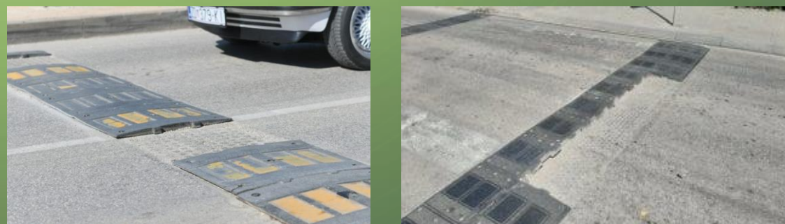
Damaged rubber elements
